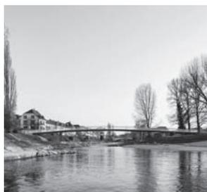
The river Birs near its estuary is a marginal location compared to the river Rhine and the close-by power plant which brand this recreational area. Therefore the new bridge is neither a suspension bridge nor an expensive framework, but rather a piece of path, a few metres of floating asphalt. The surface lifts off the ground and leads the walker, jogger or cyclist over the river on a gentle arc.
